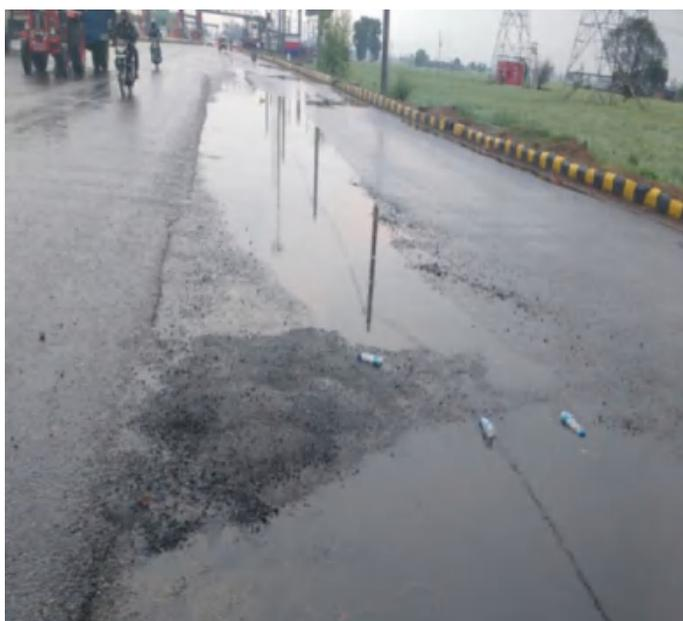
Fig. 5 Adverse slope resulting into stagnation of water on the road
