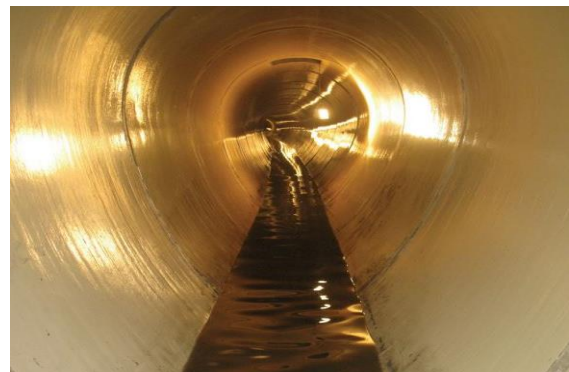
Figure 1.3: Rehabilitation of Brick Combined Sewer in Kolkata
